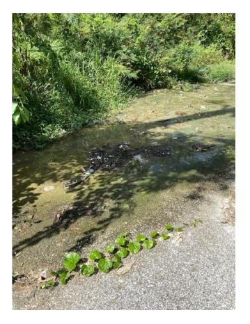
Photo 4: The sewage was flowing from the entrance manhole thru the road to a dry channel.
